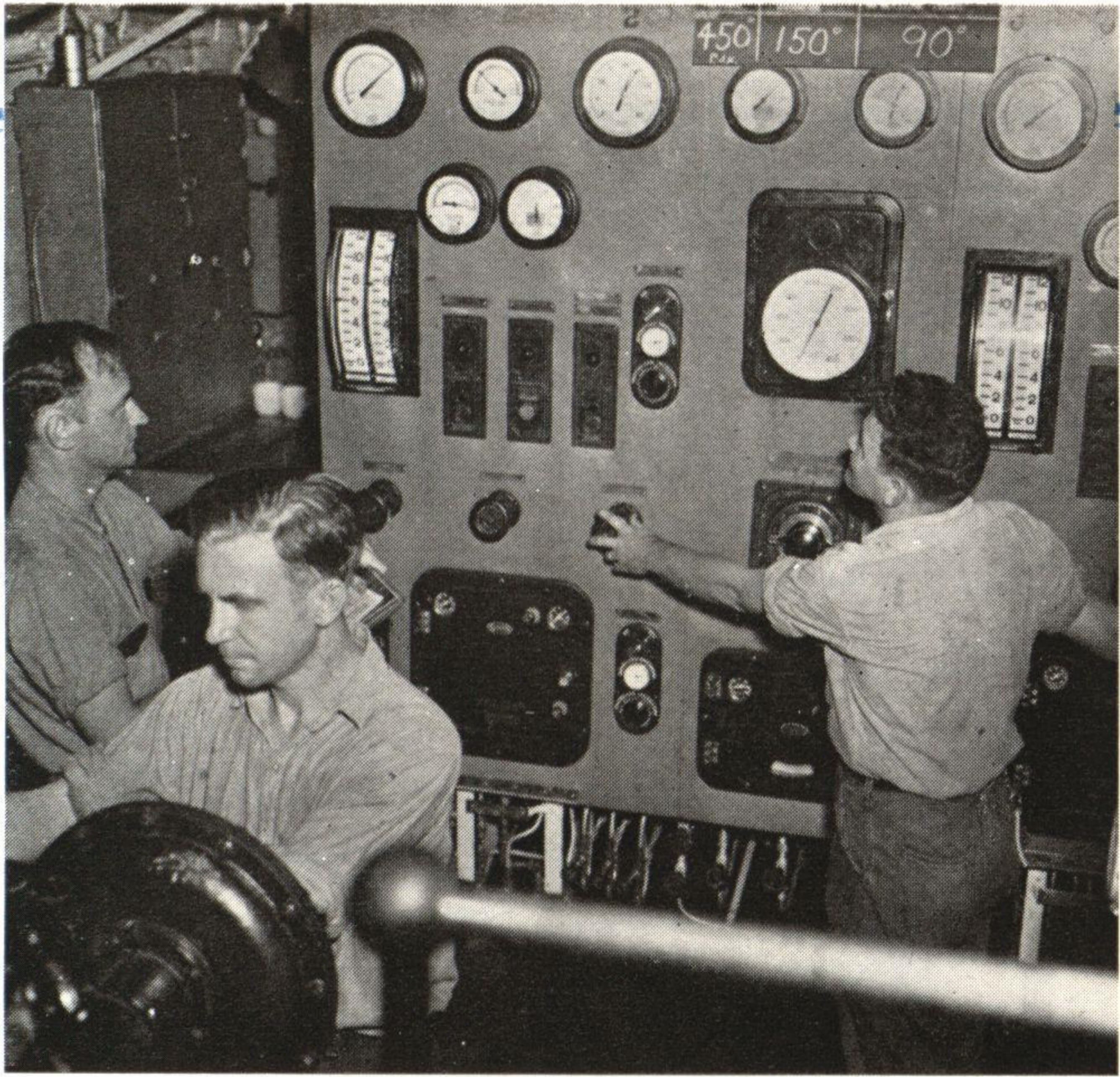
BOILER CONTROLS
